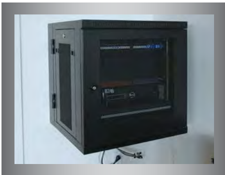
Figure 3: After Tripp Lite, physical access to equipment and media is restricted, complying with PCI requirements.
