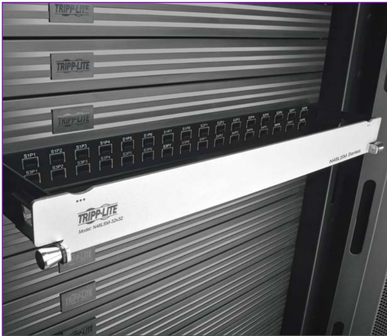
New panels require no LC-to-LC patching, double cassette or user cable shuffling.
