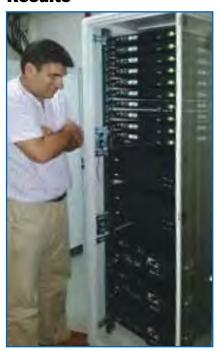
Aritech shpk, a Tripp Lite partner, provided the solution to Raiffeisen Bank Kosovo's redundancy issues. Three SMX5000XLRT3U and two SU6000RT3UHV UPS systems provide reliable battery backup power and interruption-free maintenance thanks to a hot-swappable battery. 10 PDUMH20HVAT Auto Transfer Switch PDUs provide redundancy as each is supplied by two power sources.
